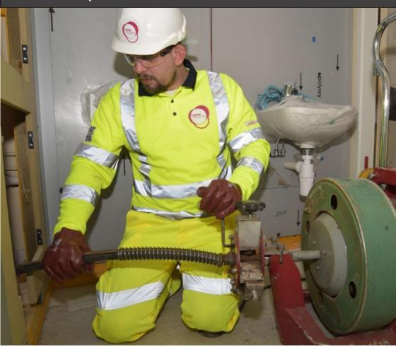
To support a £38 million refurbishment scheme at Aberdeen Royal Infirmary, Lanes surveyed and cleaned 88 combined foul and rainwater downpipe stacks, with a total length of 1,500 metres, and surveyed and cleaned 1,000 metres of underground pipework.
